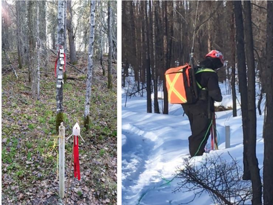
Figure 2 – Left: seismic source location: permanent buried cased holes. Right: Seismic crew loading a source location with 125g of dynamite during the acquisition campaign in February 2021.
